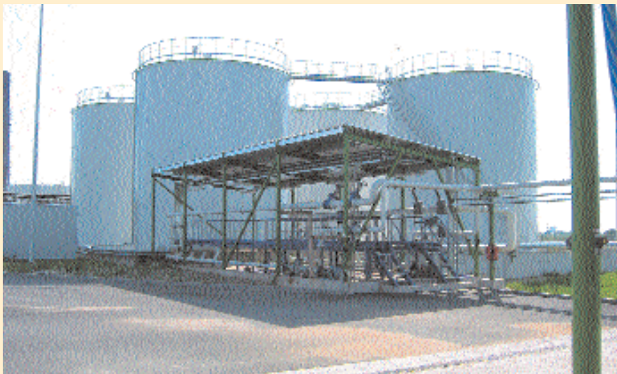
NCC&PO: New extension of the terminal completed in 2003.
